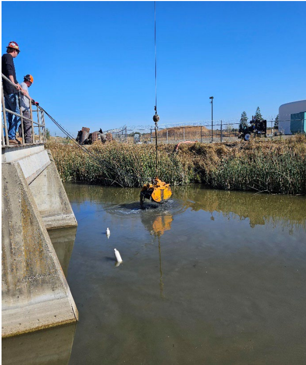
Dredging soil in front of Main Pump Station
