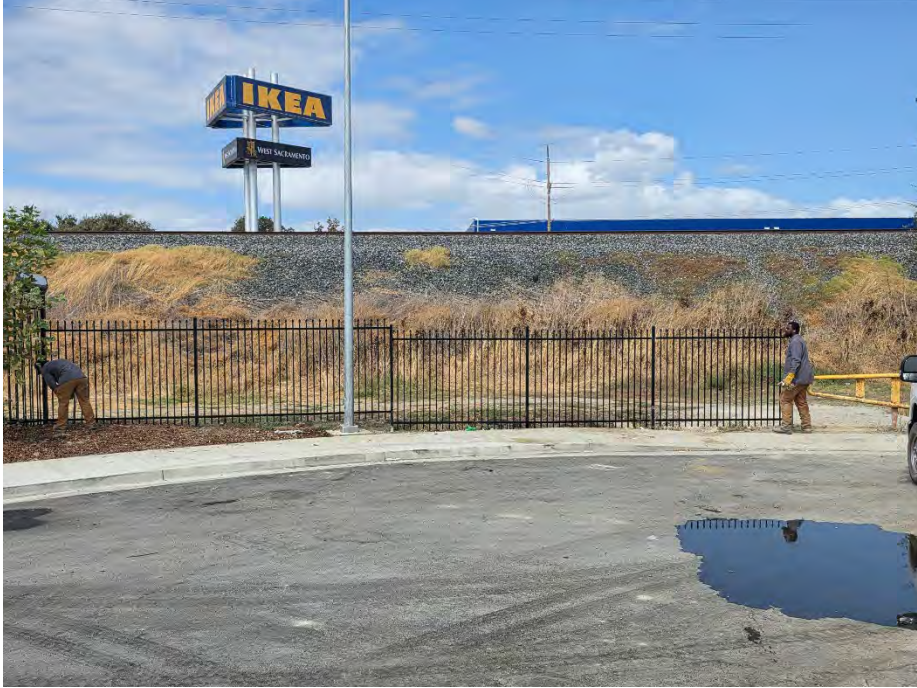
Fence installation on Sutter St.
