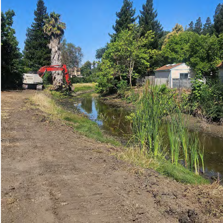
Blacker Canal – tree/vegetation removal
