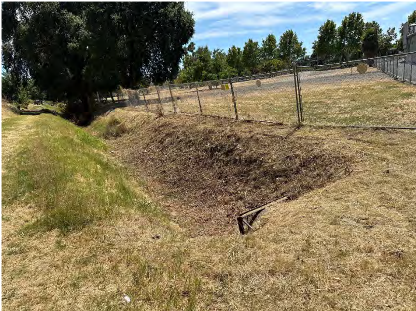
Ditch behind Bowling Alley - cleared
