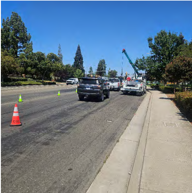
Blocking traffic to remove tractor
