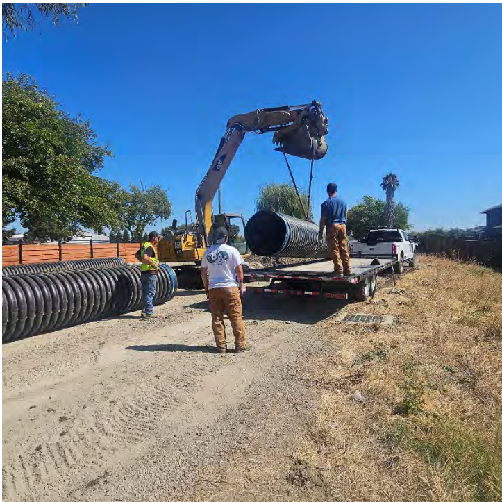
Unloading culvert near Parella Estates
