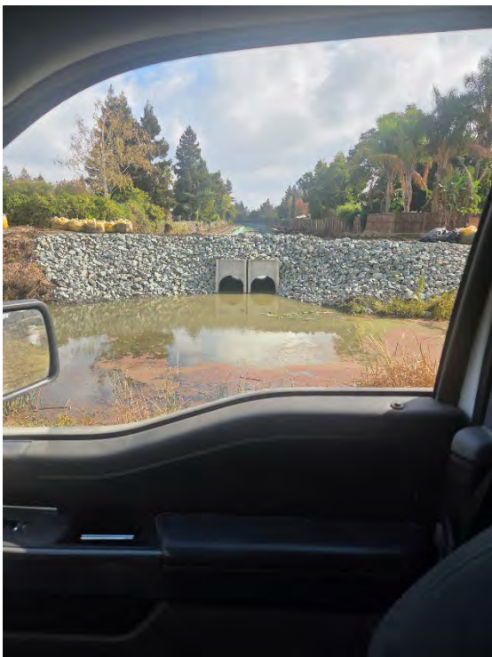
Blacker Canal at Main Canal, new crossing
