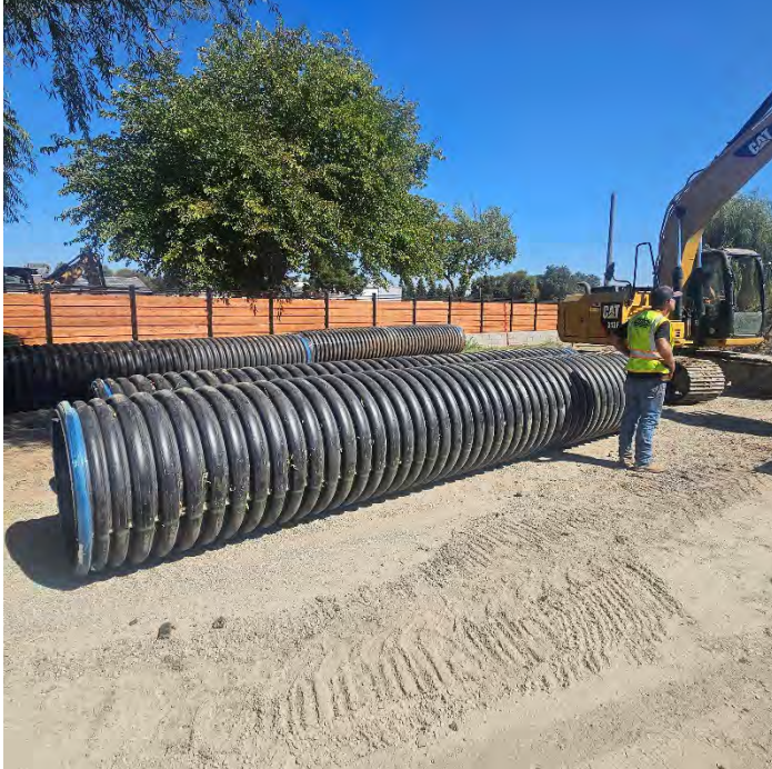
Installing storm culvert near Parella Estates
